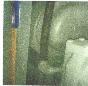
Modified Design (With Elbow & Nipple fitting)
