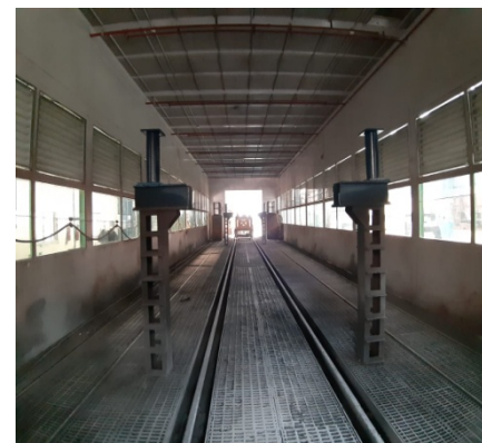
Modified Paint booth
